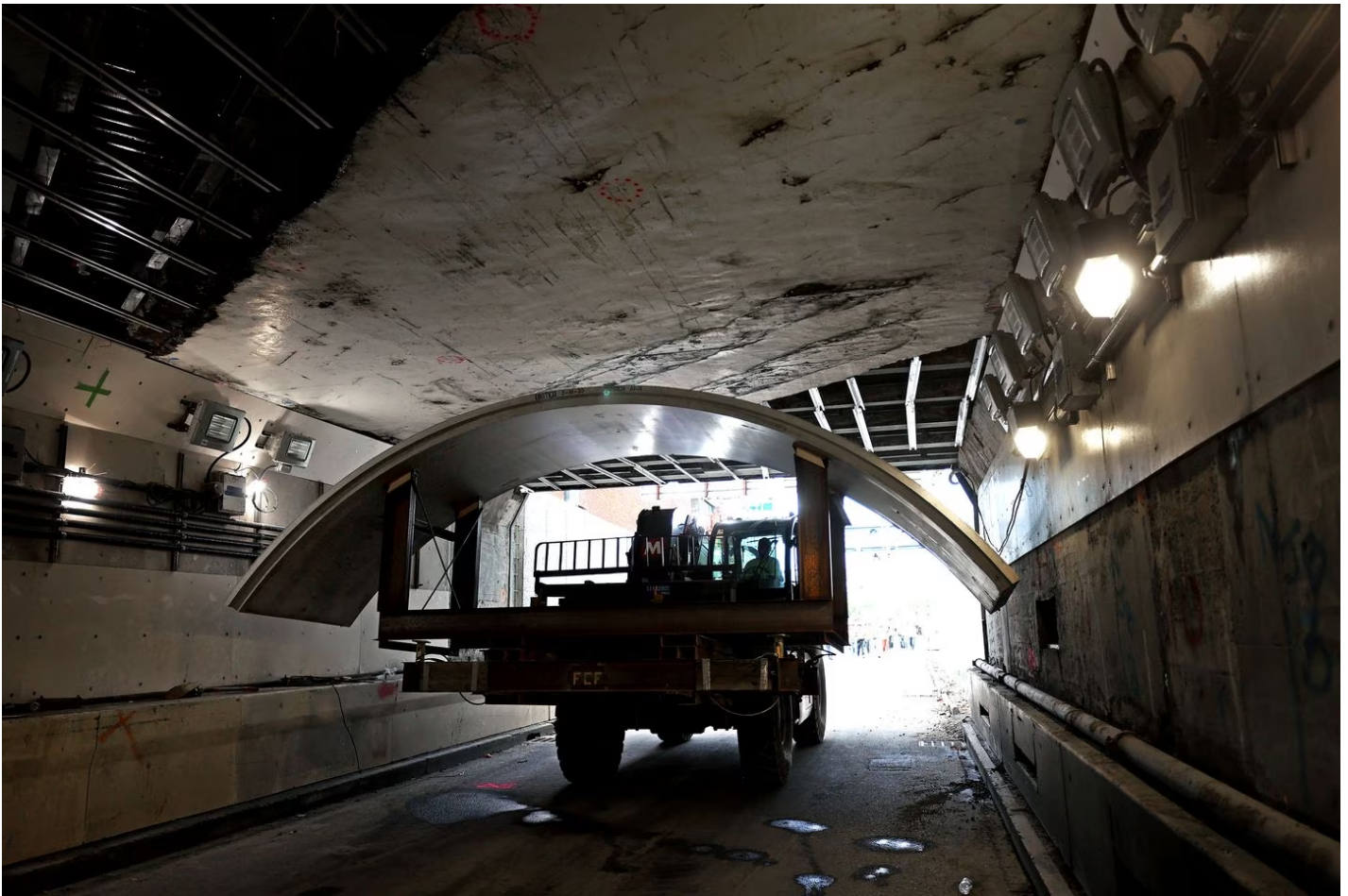
A curved pre-fab ceiling tile made its way into the tunnel on a machine similar to a giant forklift. DAVID L. RYAN/GLOBE STAFF
